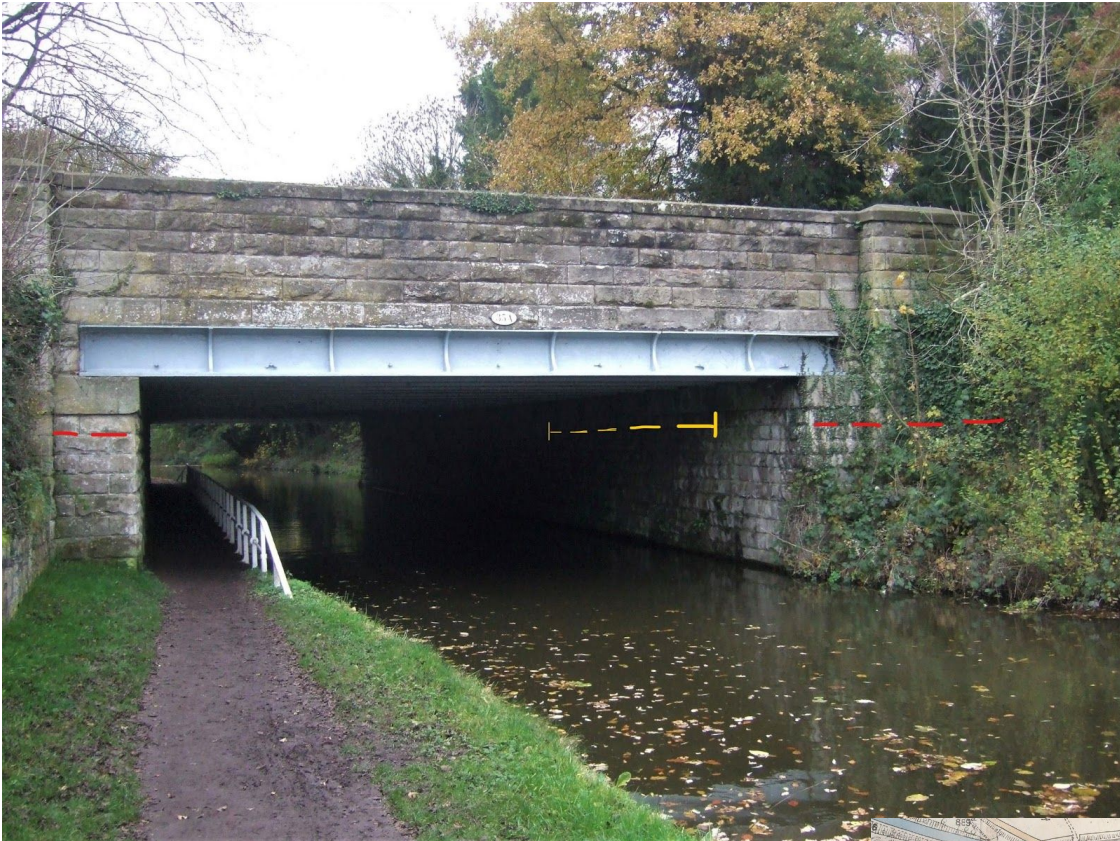
9. Closer view: The best estimate of the location is shown by the dashed yellow line. The red line is the estimate of the original ground level before the canal.
