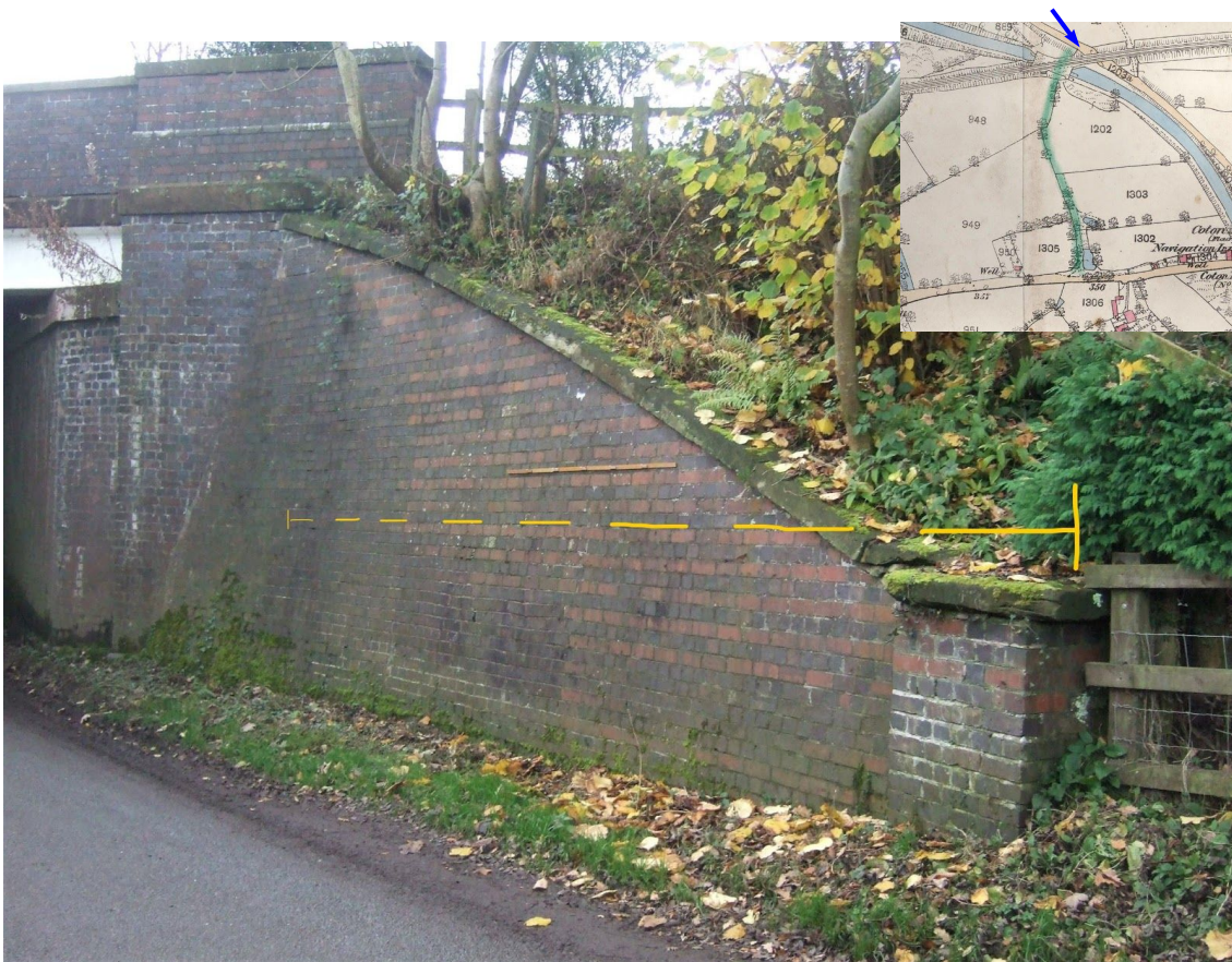
12. Closer view of the junction as it looks in 2020. The 2m long rule (above the yellow line) is set at the ground level in the field opposite. The surface level of Gill Brook Lane would have been somewhat lower due to erosion through usage.
