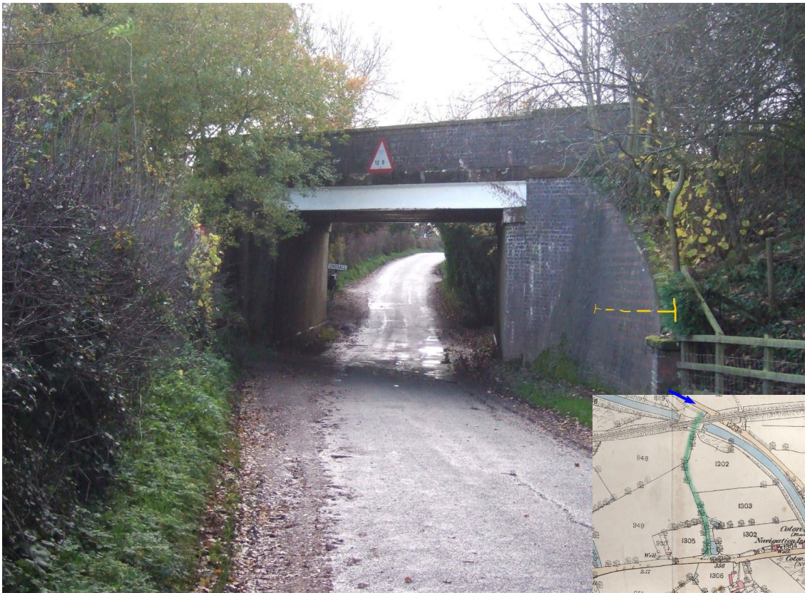
11. Location of Plardiwick Lane and Gill Brook Lane junction. Plardiwick Lane has been deepened by about 2m to create sufficient headroom for the railway bridge.
