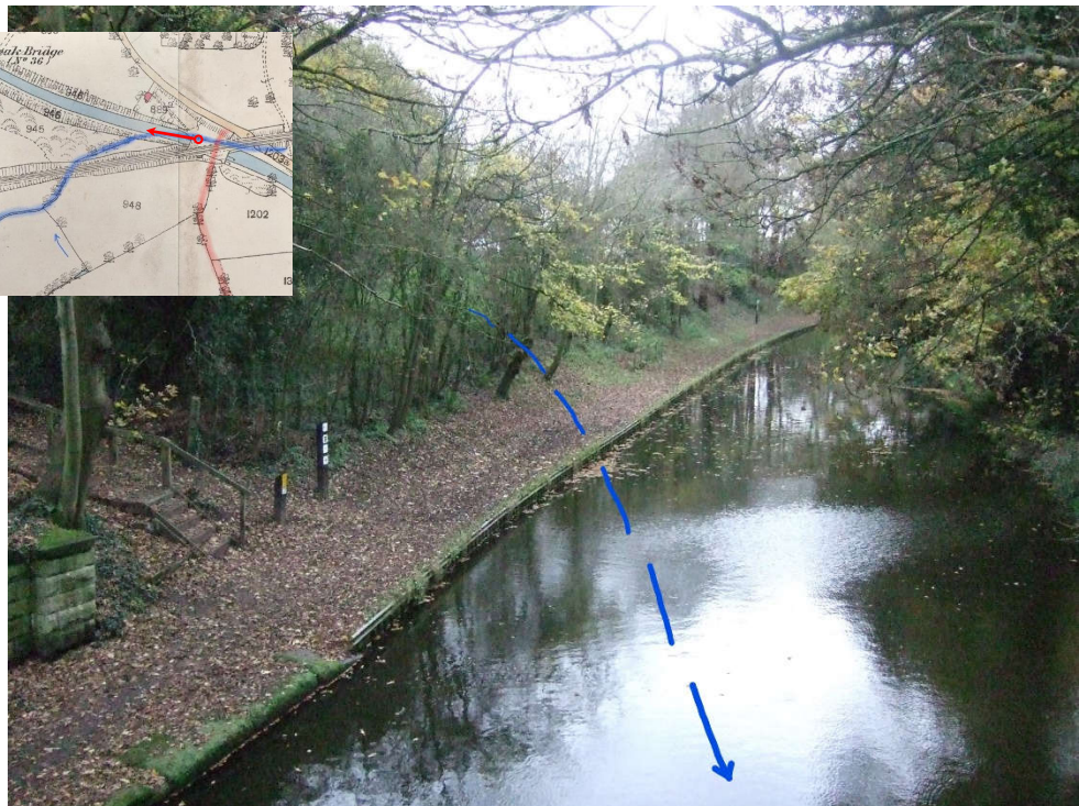
8. The blue line is a best estimate of the original course of Gill Brook before the coming of the canal, necessitating its diversion.
