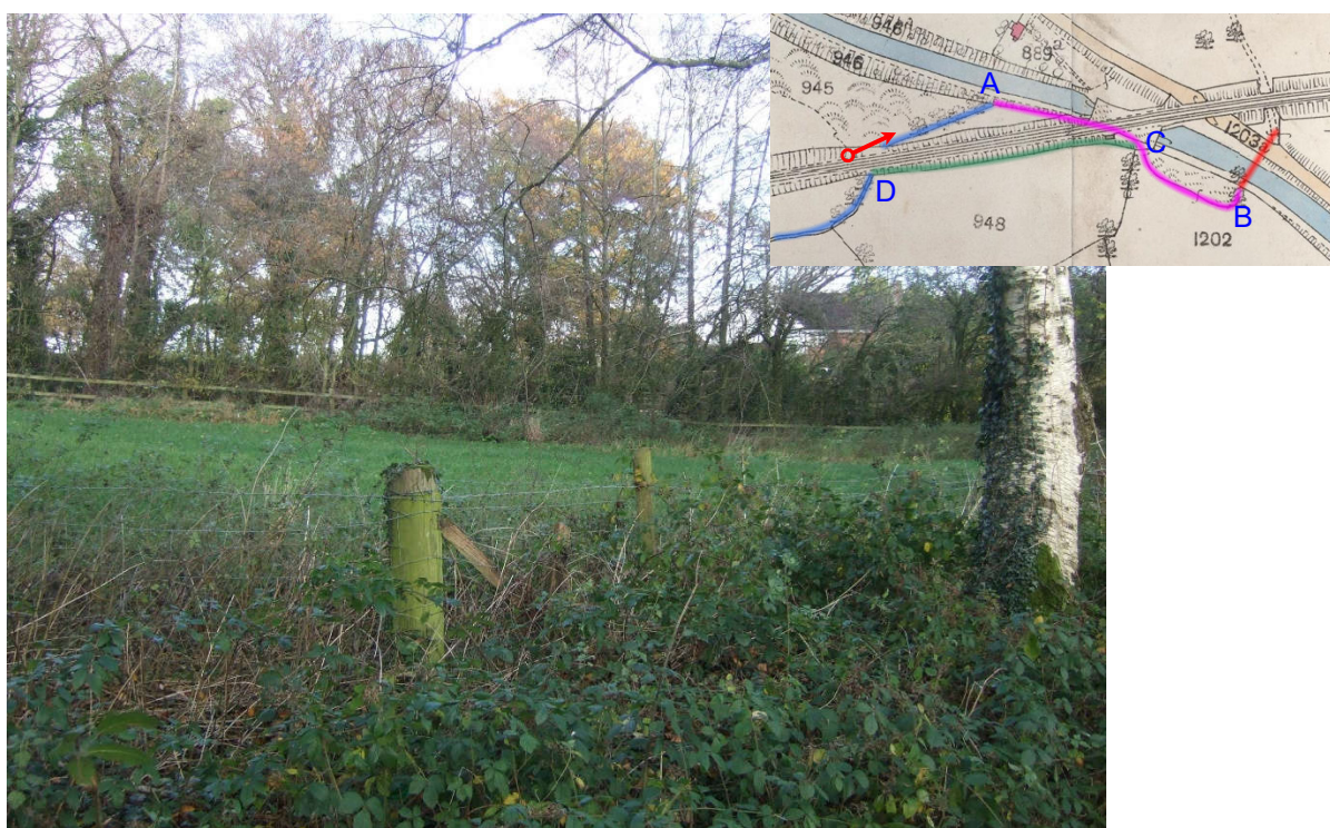
10. Downstream view: D to A. There is no trace of any watercourse. The fence in the middle ground marks the top of the canal cutting. Plardiwick Manor Cottage is just visible through the trees on the far bank of the canal.
