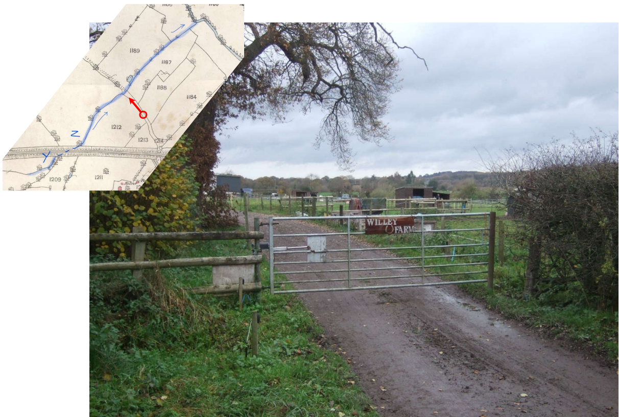
34. Gill Brook is piped under Willey Lane just in front of the gate.
