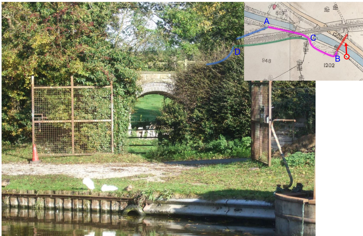
21. The culvert was built on a steady gradient passing under the canal and Plardiwick Lane to discharge into a 5m deep chamber between the lane and the bridge.
