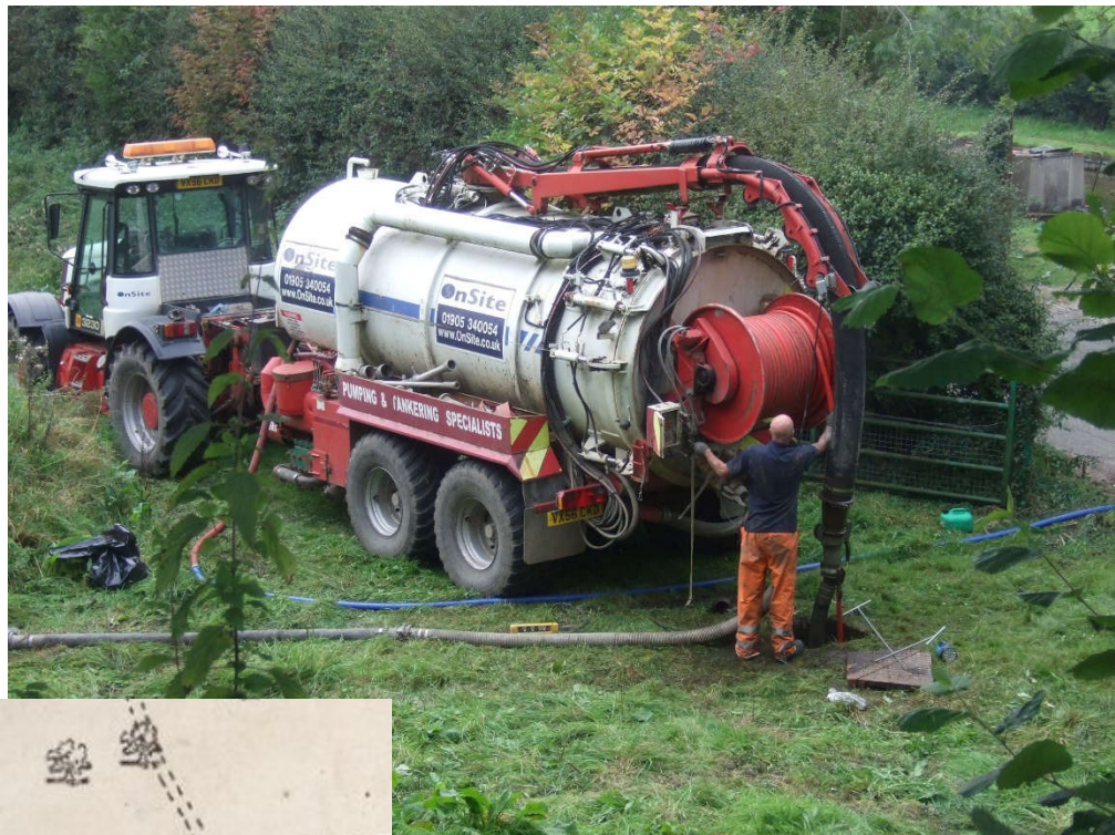
22. The Canal and River Trust's contractors cleaning silt out of the chamber and culvert in September 2020. It took them 4 days to complete the work.
