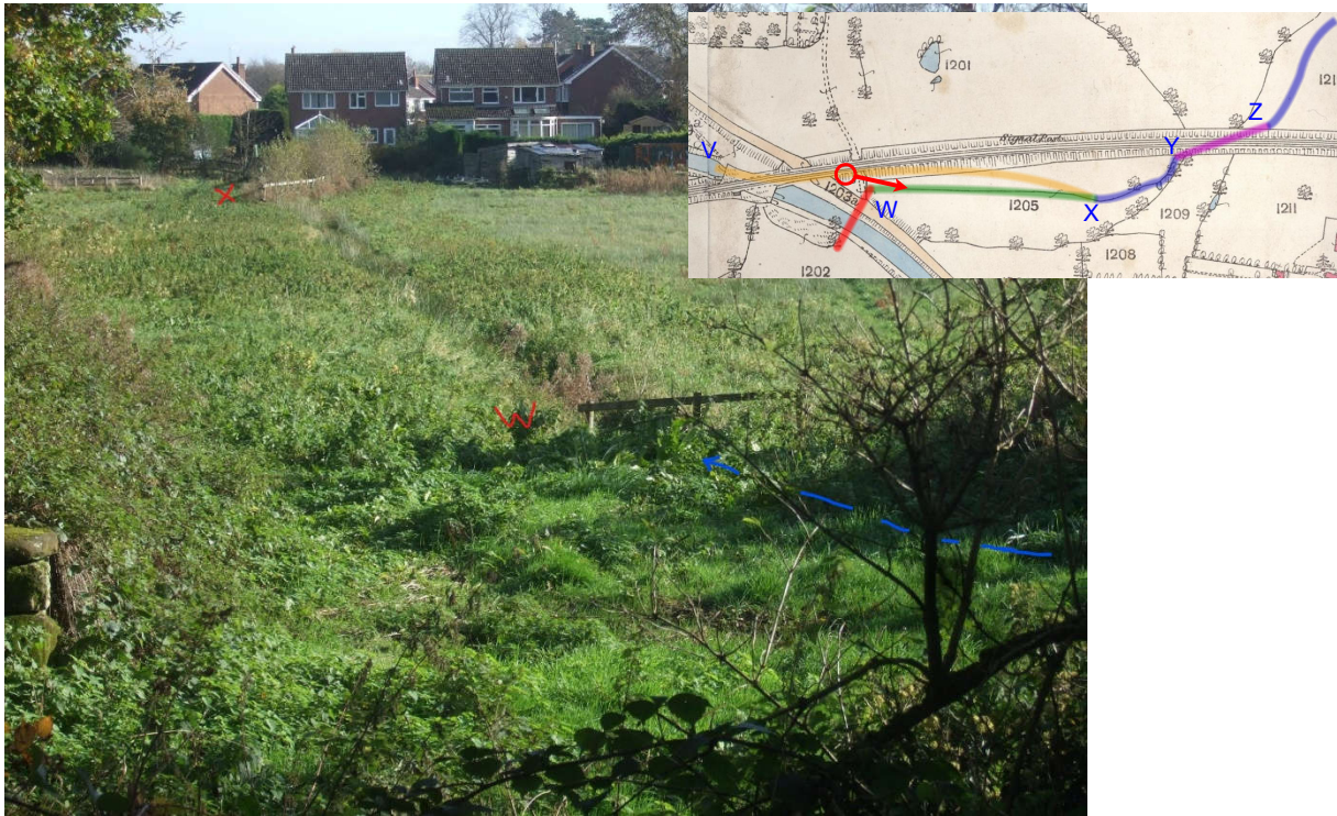
24. Taken from the steps of Plardiwick Lane Railway Bridge looking toward Glendower Close. The broken blue line maps the route of the outfall from the chamber to the open channel (drain) at W. At X the channel picks up the original course of Gill Brook.
