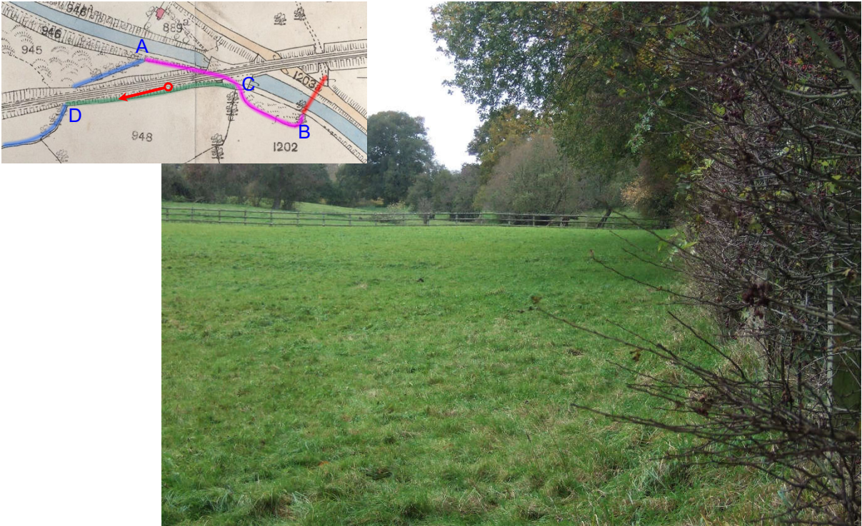
13. Shows the Post and Rail Fence with Gill Brook beyond it. The pipe installed by British Railways pipe is about 0.5m into the field and parallel to embankment, and has made a significant improvement in the surface quality of the field.
