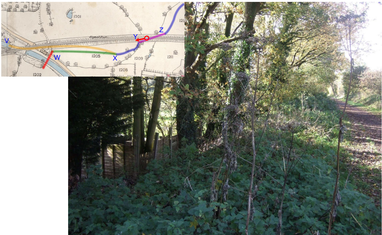
27. Taken from the railway looking upstream in the vicinity of the culvert Y – Z. The back gardens of Glendower Close are on the left.
