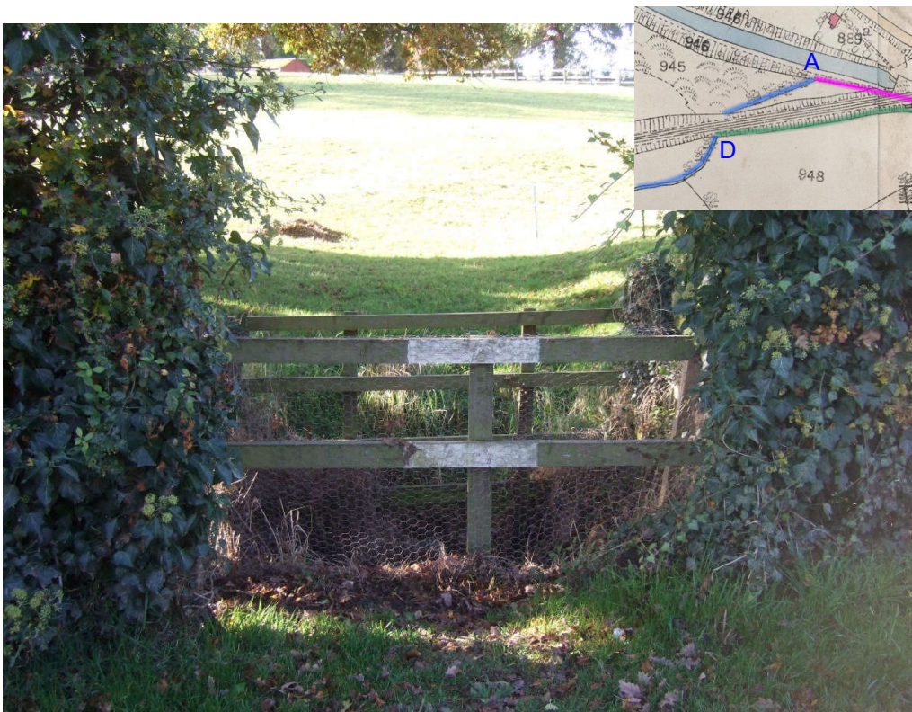
19. Culvert access shaft and safety fencing.
