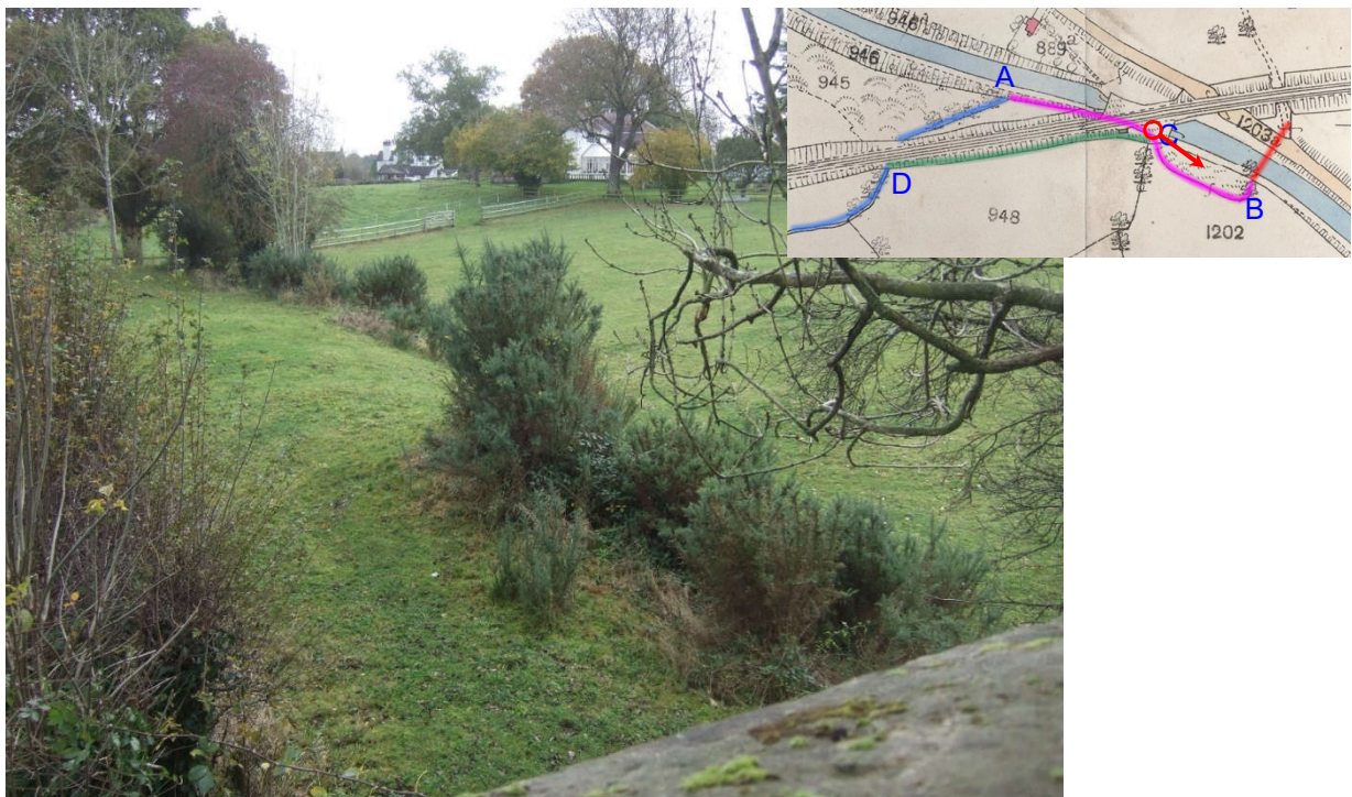
16. Taken from the parapet of the railway bridge. The gorse is growing on what was once a spoil mound formed when the canal was first dug. The diversion flowed in an open ditch along the side of this mound before looping around the end of it to enter the culvert under the canal at point B, but the ditch has now been piped.
