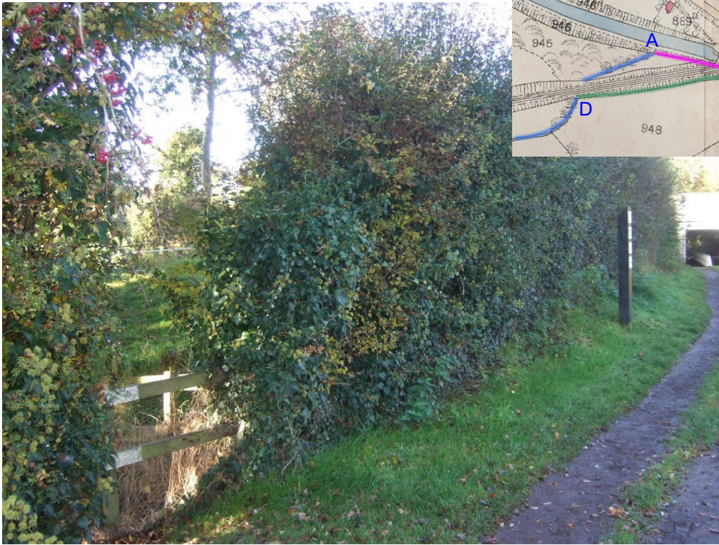
18. This view shows the location of the culvert in relation to the towpath and bridge.
